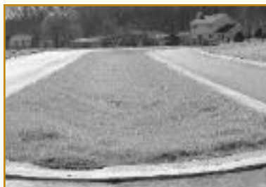
Below: Thermal swale, designed to absorb runoff in an urban area.
