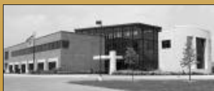
Dane County's Fen Oak Resource Center, home of the Land Conservation Department
